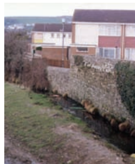
THE OLD SEA WALL AT WRAFTON
